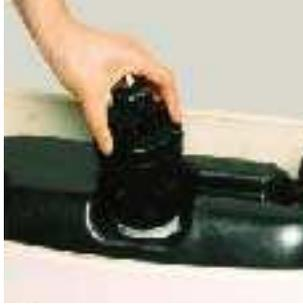
Step 9. If the tank continues to run, remove the FVC and check that the lower piston is in the proper position and check the large o-ring to ensure that it is properly seated. When the vessel is filled and the water stops running, it is an indication that the vessel is filled and ready to continue normal use.
