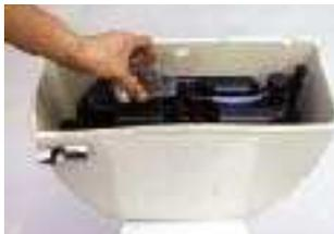
Step 5. Check the Flush Valve Cartridge (FVC) for air leaks by pouring a small amount of water onto the area around the top of the flush valve cartridge. If air bubbles are visible then you must remove the FVC and check the flush valve o-ring for damage and to see that it is properly positioned in the vessel. If air bubbles are observed then you must remove the Flush Valve Cartridge and inspect the o-ring for damage and proper seating.
