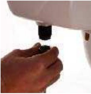
Step 3. Check to ensure that there are no kinks in the supply lines or connector lines between lower and upper supply assemblies, which would prevent the flow of the water into the system. Also check that there are no leaks at any of the connections.
