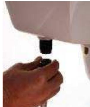
Step 2. Check for debris in the filter screen system at the water inlet for any obstruction that might limit the flow of water into the vessel. To do this shut off the water supply, flush the unit to relieve any pressure and disconnect the water supply line from the threaded connector. You can remove the filter screen easily using a set of long nose pliers. Clean and replace the filter screen. Then reconnect the water supply and check the water flow.
