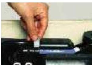
Step b. Remove the quick connector line between the Upper Supply Assembly and the Flush Valve Cartridge by rotating the locking tab downward. Remove the supply line and set it aside.
