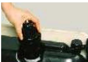
Step d. Remove the Flush Valve Cartridge (FVC) Assembly using the tool provided. Using the FVC tool, engage the teeth of the tool with the slots on the top of the FVC and with the aid of wrench, rotate the FVC counter clockwise  $\frac{1}{4}$  turn, then lift the FVC up removing the FVC and the upper o-ring. Inspect the upper o-ring and the flush valve seat of the Flush Valve Cartridge.
