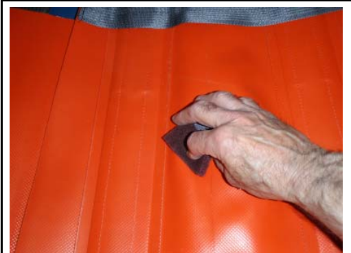
Clean and apply masking tape on the backside of the tear.
