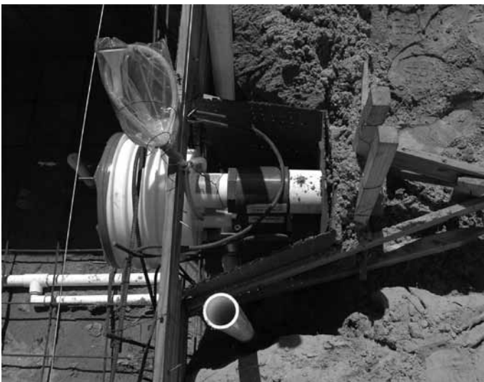
Fig. 7 Setting the BADUJET housing into reinforced steel
