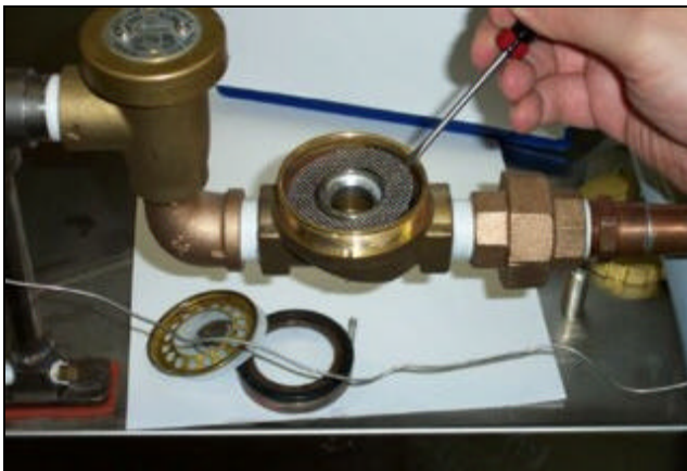
Removing the mesh strainer screen
