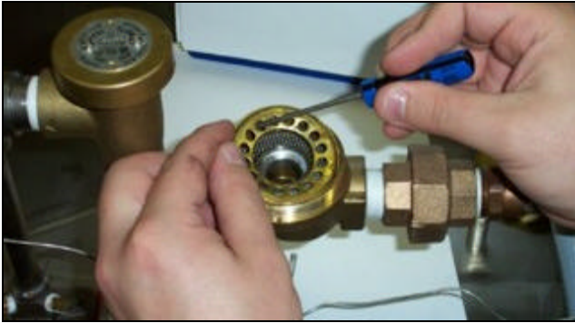
Removing the screen retainer
