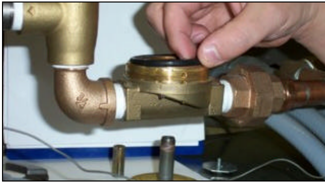
Removing the O-ring
