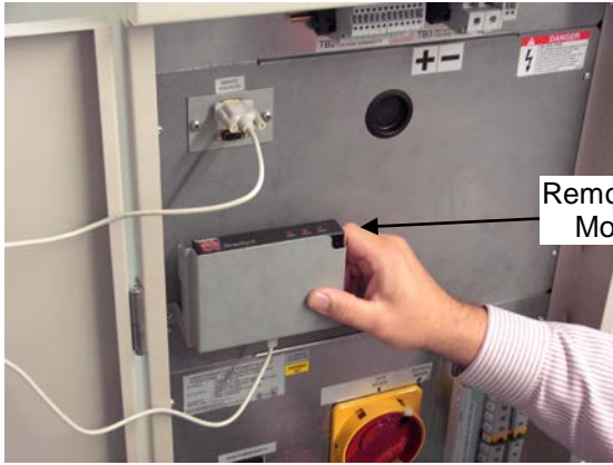
RemotEye II Mounting Location – 15-30kVA
