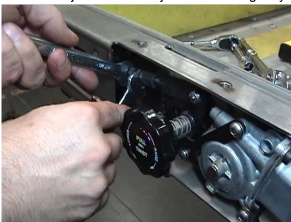
FIGURE 4-11: LOOSEN JAM-NUT
