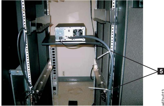
*Figure D-2. Rear view of shelf with cables attached to rack rails with tie wraps*
