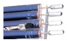
Prepare the tubes for inserting into the collector manifold, coat a thin layer of heat transfer paste over the condenser part of the heat pipe. After this apply soapy water to the tube ends a shown in the picture.
