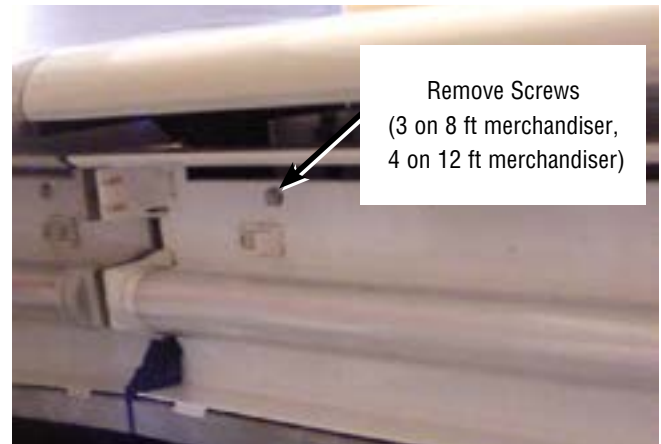
Remove Front Lamp Assembly to Access Screws
