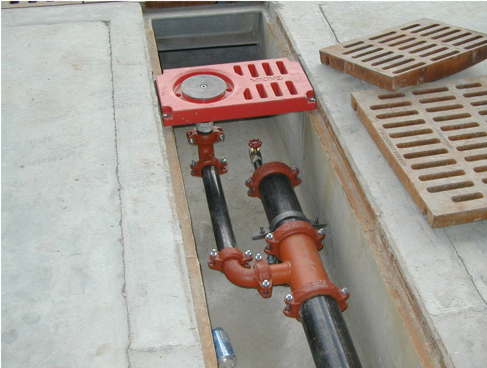
Figure 2 Typical Low-Level AFFF System Piping
