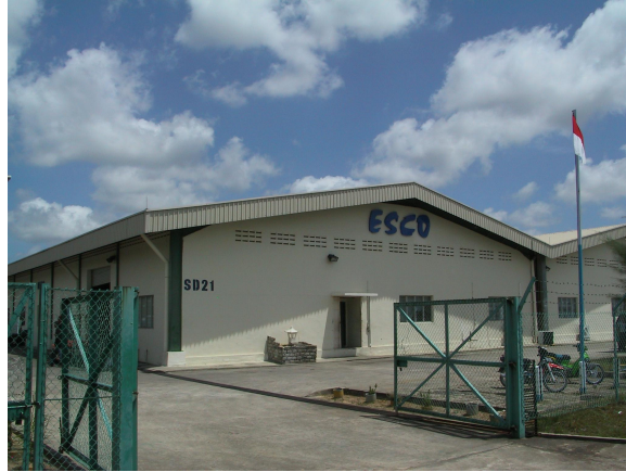
Fig. 2 Esco Production Facility
