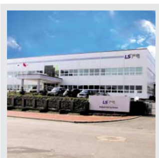
Dalian Plant (China)
