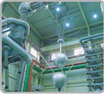
High Voltage Test / Impulse Test
