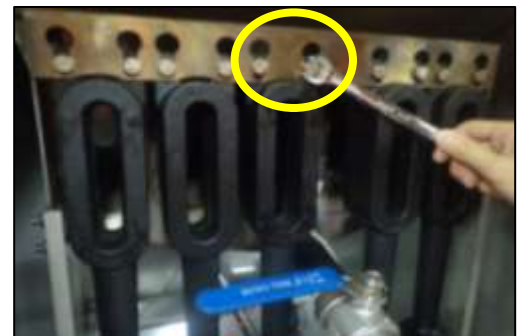
Loosen the two mounting screws of the burner
