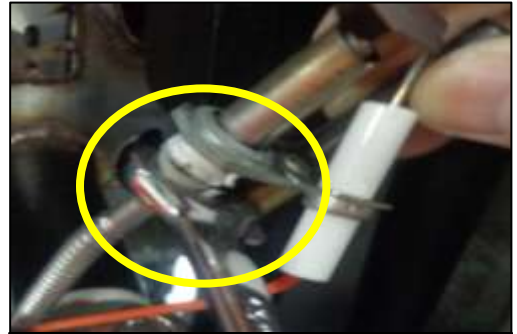
Disconnect the pilot tube from the FDS assembly
