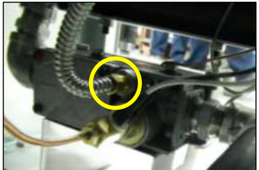
Disconnect the pilot tube from the combination valve
