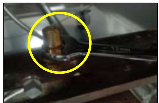
Remove the burner injector from the manifold
