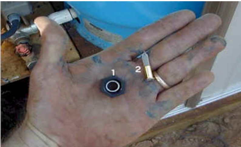
Brine Tank Photo #2
