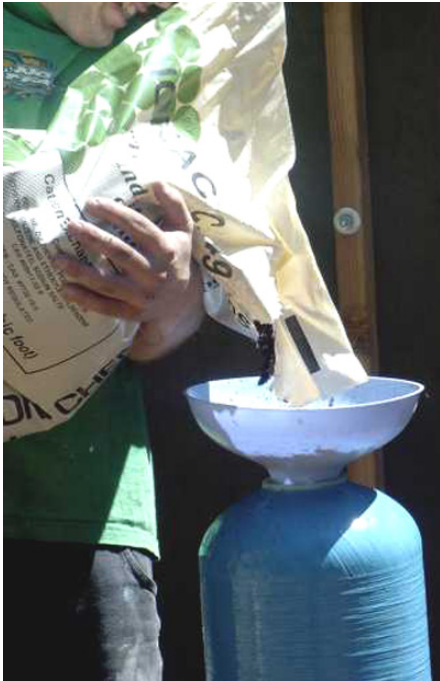
Adding resin to the tank.
