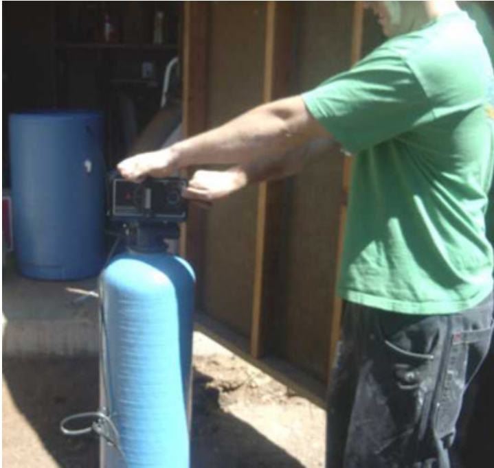
Skrewing valve onto tank.
