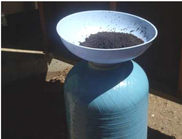
Adding resin to the tank.
