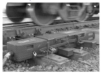
The ECC utilizes inductive proximity sensors to continuously monitor switch-machine conditions. It vitally monitors the position of the switch points and the internal locking mechanism, delivering switchmachine indications to the wayside.
