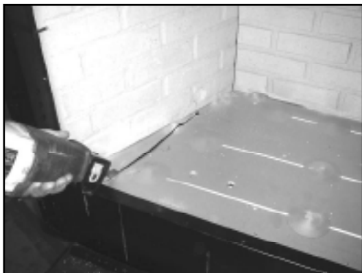
Figure 11.2. Using a saws-all, cut out the floor.
