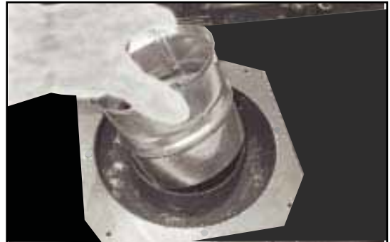
Figure 8.2 Remove the inner collar adapter.
