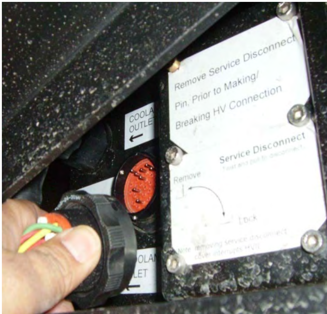
Figure 34: Removing the LV connector from ESS (HV Battery)
