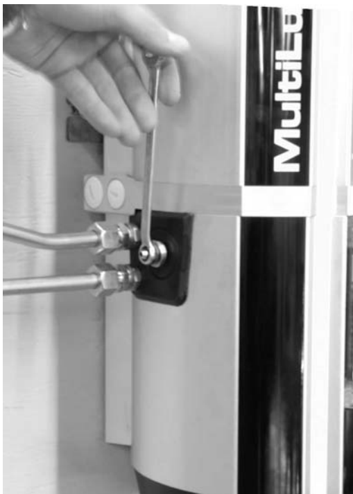
Figure 1. Opening the deaerating screw
