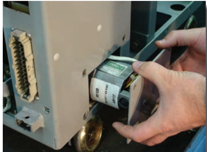
Figure 11 Removing the Charging Motor from the PowlVac-ND Circuit Breaker
