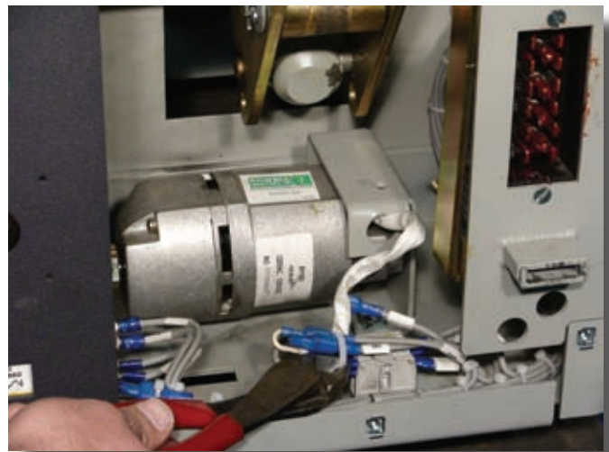
Figure 2 Cutting the Tie Wrap
