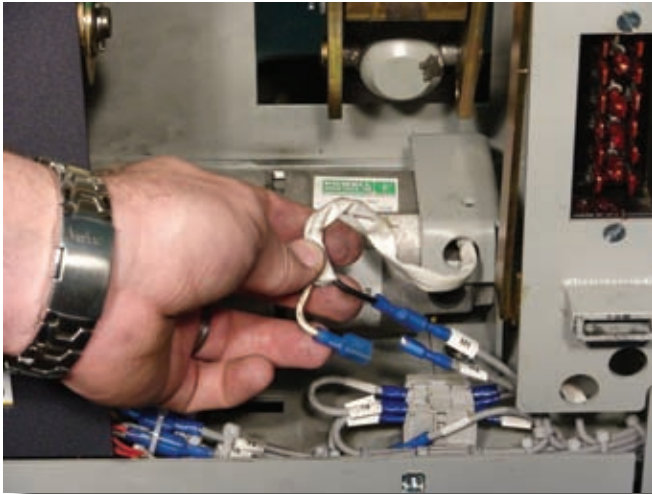
Figure 3 Disconnecting Charging Motor Wires from the Wiring Harness
