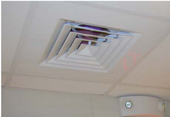
HVAC Vents Discharge
