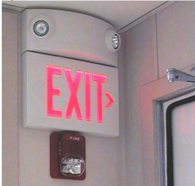
Figure 53: Emergency Dual Beam Lighting
