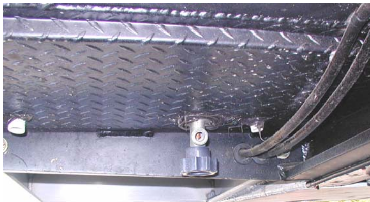
Figure 41: Humidifier External Water Connection
