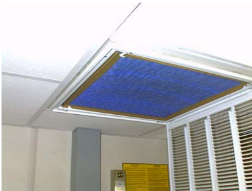
Downstream Blower Filter Access
