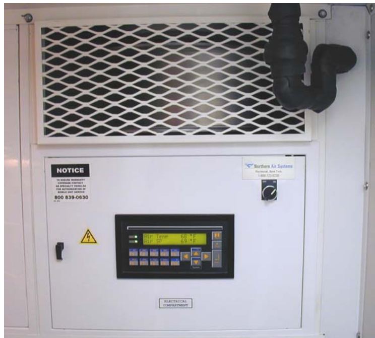
Figure 44: A/C / Chiller Control Panel
