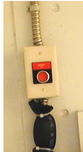
Emergency Off Button, Magnet Room
