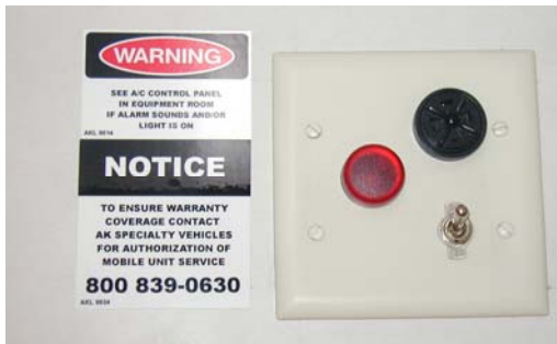
Air Conditioning Trouble Light & Alarm
