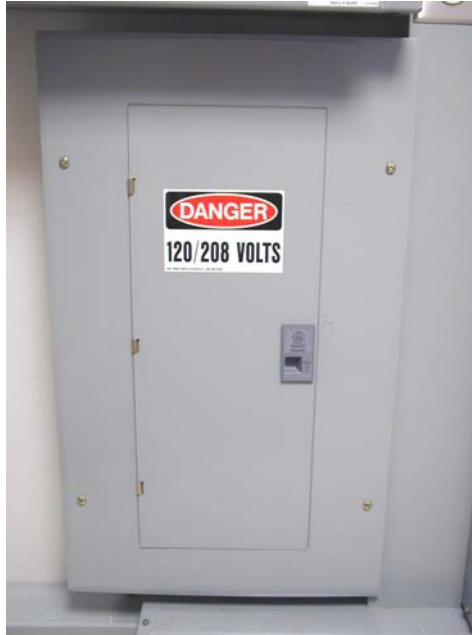
Figure 33: 120/208V AC Electrical Panel
