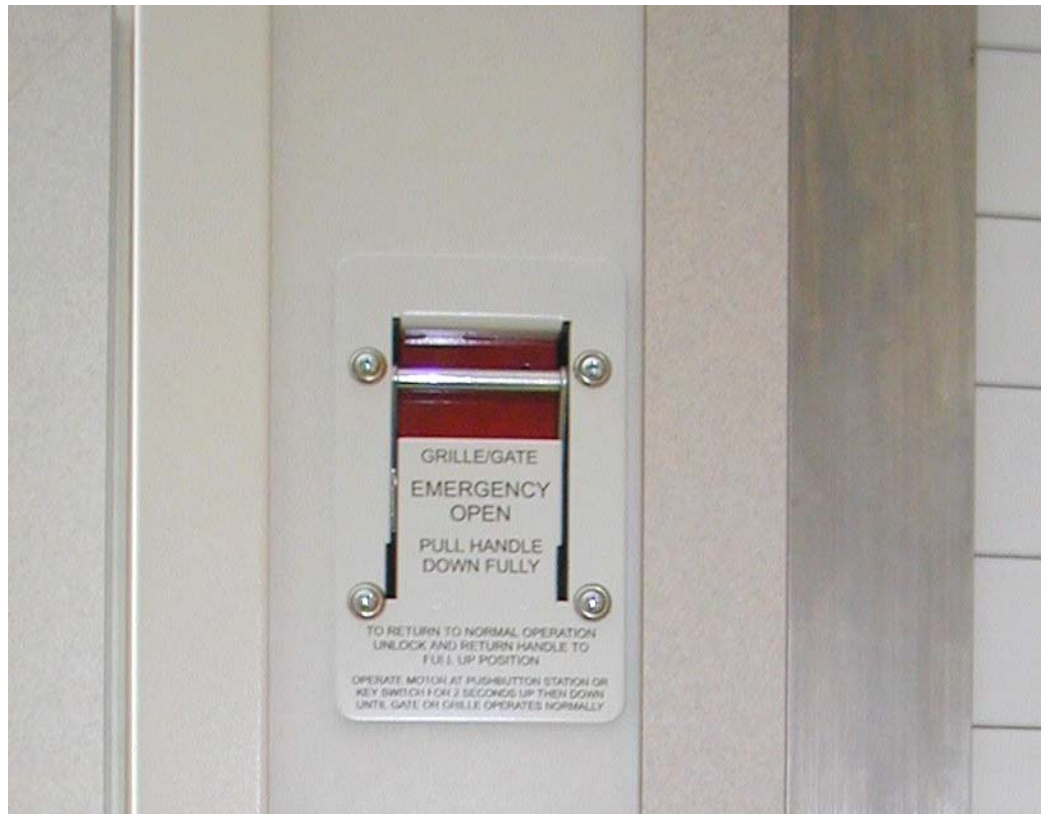
Figure 31: Roll Door Emergency Release
