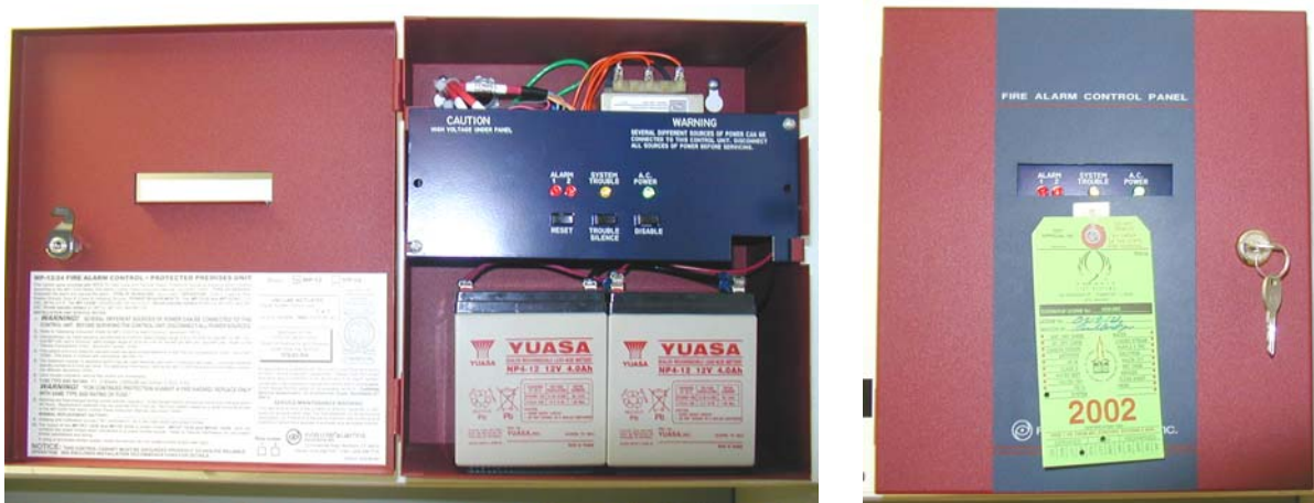
Figure 26: Fire Alarm Control Panel
