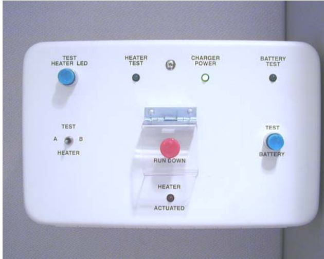
Guarded Magnet Quench Button, Scan Room
