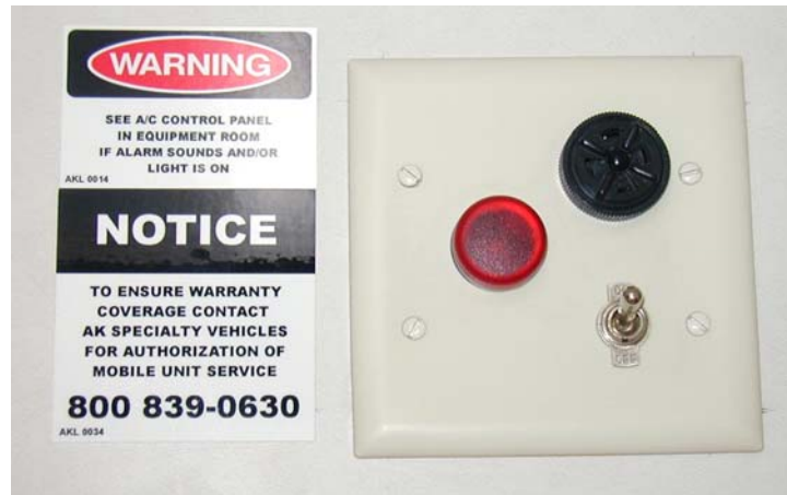
Figure 45: A/C / Chiller Alarm Panel
