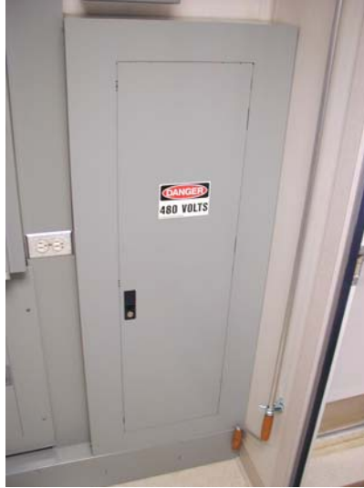
Figure 34: 480V AC Electrical Panel
