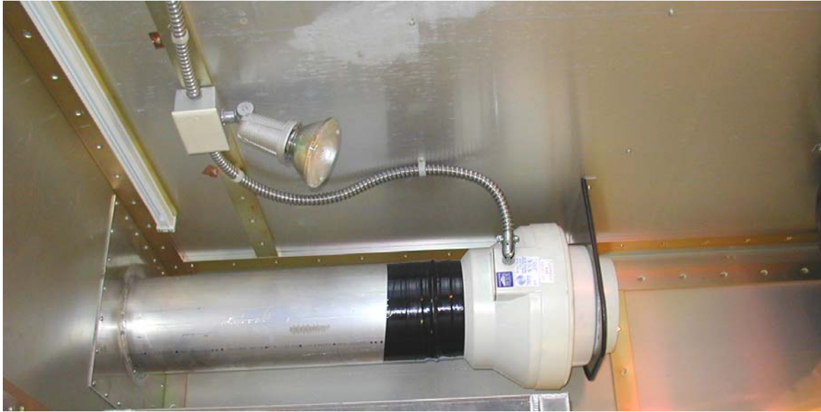
Figure 14: Magnet Room Helium Gas Exhaust Fan
