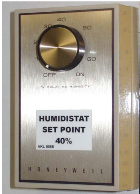
Figure 42: Humidity Controller
