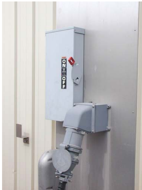
Figure 36: Shore Power Connection
