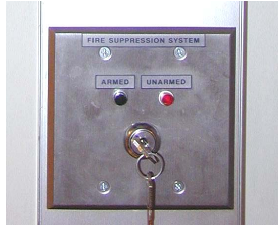
Figure 30: Maintenance Switch
