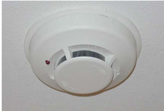
Figure 25: Smoke Detector
