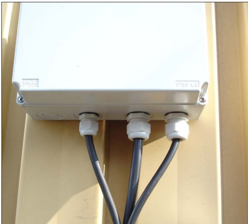
Fig 7.2.B - Wind-sensor, motor/switch, and power cable in TAC3 installation box
