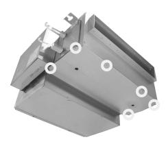
(3) Remove the LEV driving motor using two spanners. (Fig. 10) Fig. 10
