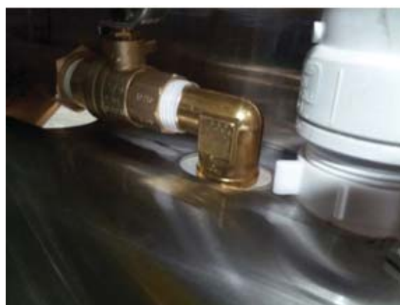
Hot water inlet at ½" elbow
