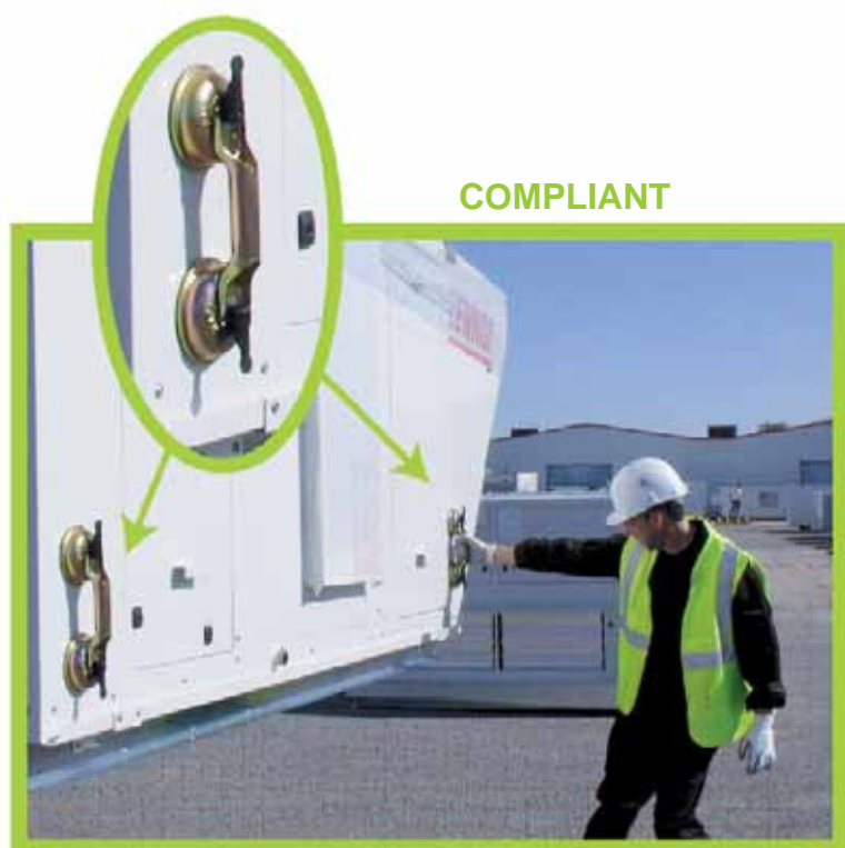
Vacuum lifting beam to position the unit
