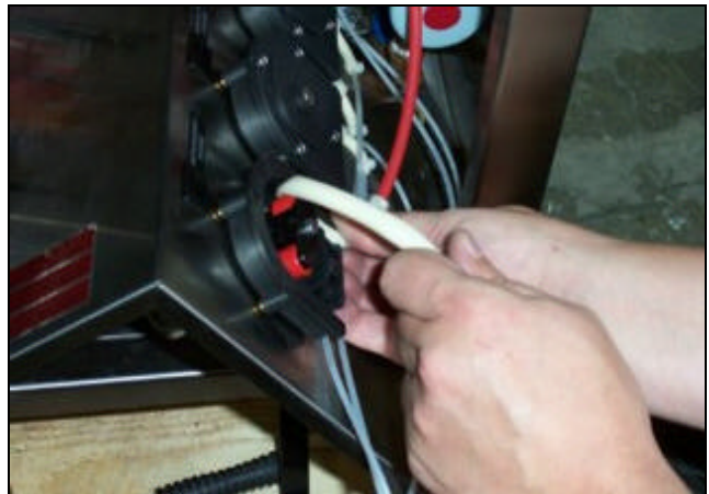
Pulling the rubber tube out of the pump.
