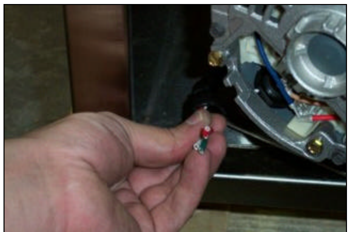
Removing the power wires.
