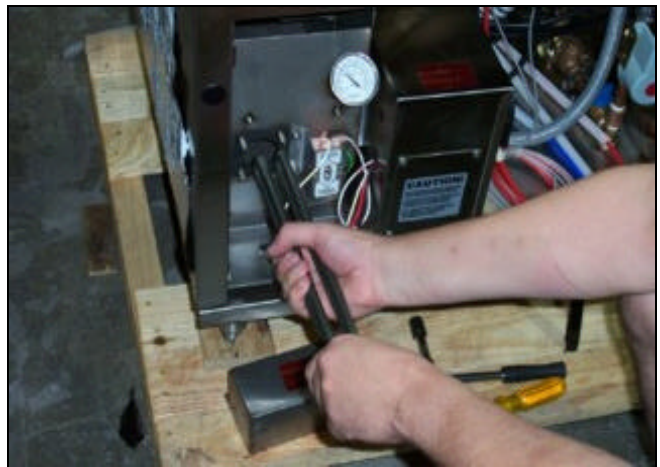
Pulling the heater out.
