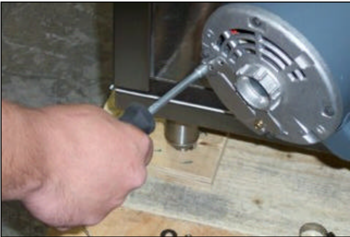
Removing the wiring cover.
