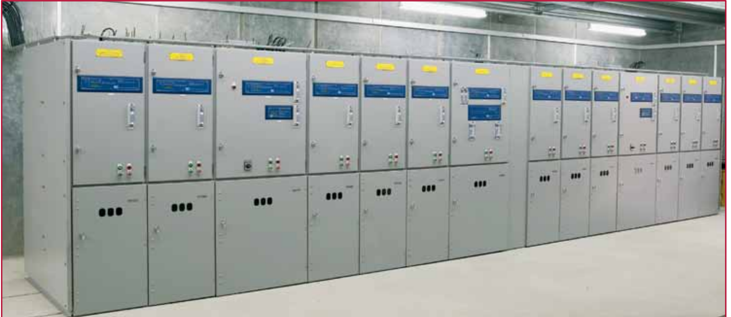
LMVP Switchboard Installation: Powerco – Main St Substation
