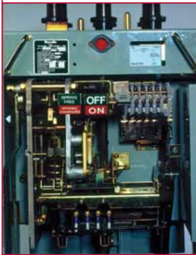
Hand charged spring mechanism – cover removed. (Type QM, X Series circuit-breaker.)
