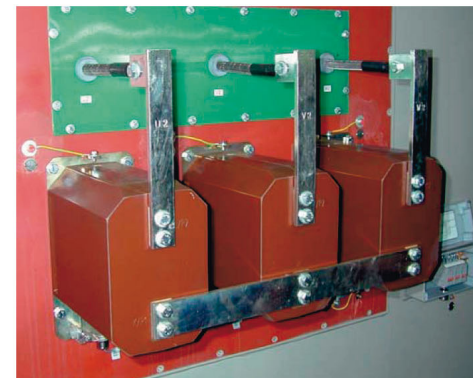
Connecting box, with outgoing star point with current transformer for differential protection
