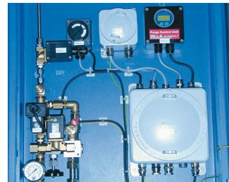
Scavenging air control system (EEx p)
