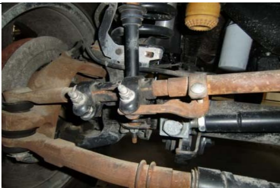
Tighten up hardware and replace keeper bolt
