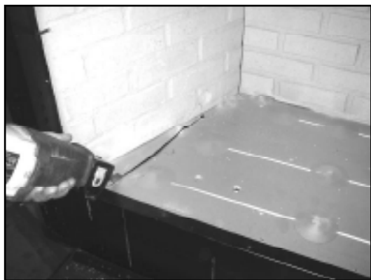
Figure 10.2. Using a saws-all, cut out the floor
