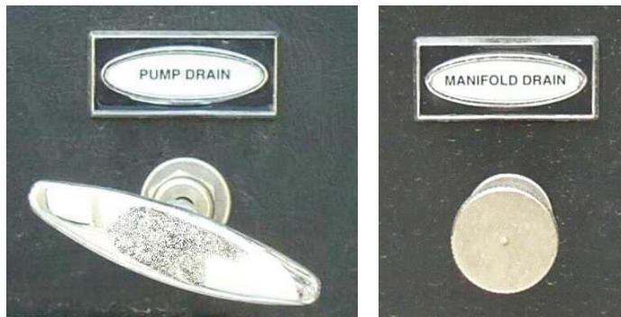
Figure 4-1: Typical Master Pump Drains
