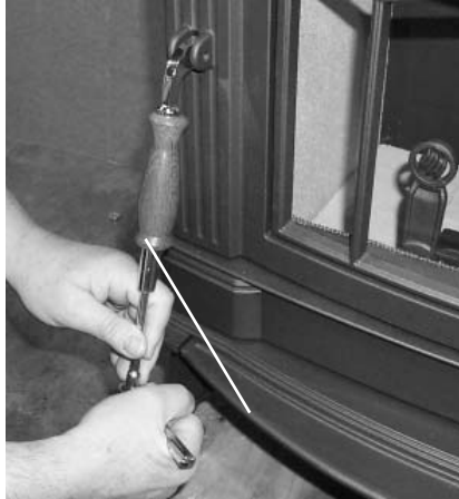
Secure using 7/16" socket wrench.
