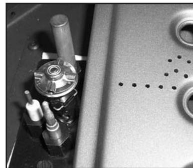
Figure 15: Burner to pilot hood relationship.
