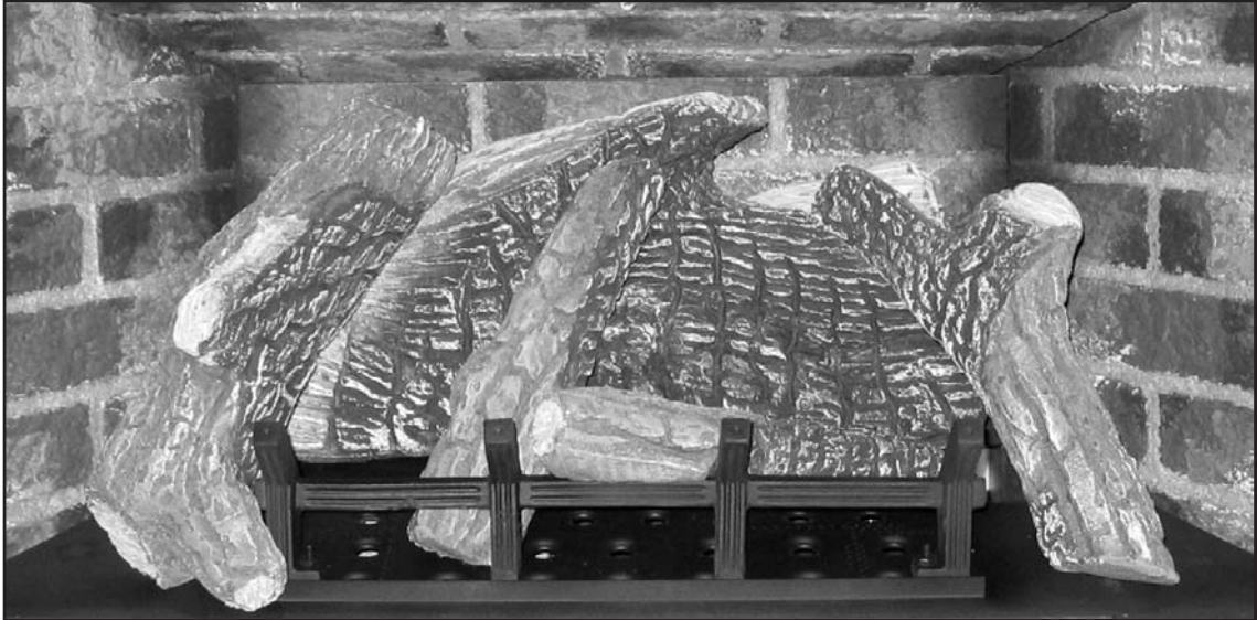
Figure 34. Third Stage Log Set Installation.
