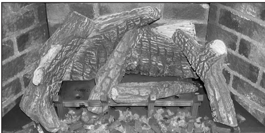
Figure 36. Fifth Stage Log Set Installation.
