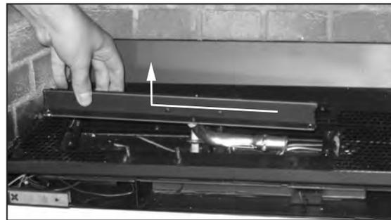
**Figure 20: Burner Removal.**
