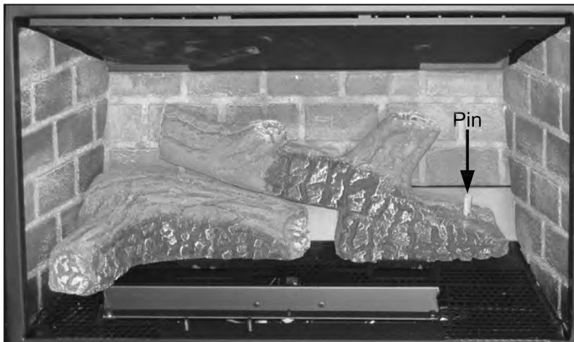
Figure 72. Second Stage Log Set Installation.
