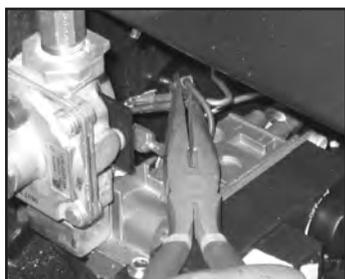
**Figure 32: Remove Jumper From Thermocouple.**
