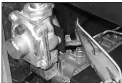
**Figure 33: Spill Switch Wires Connect to Thermocouple.**
