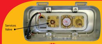
Turn to the left (Anti-Clockwise) to turn LPG supply ON
