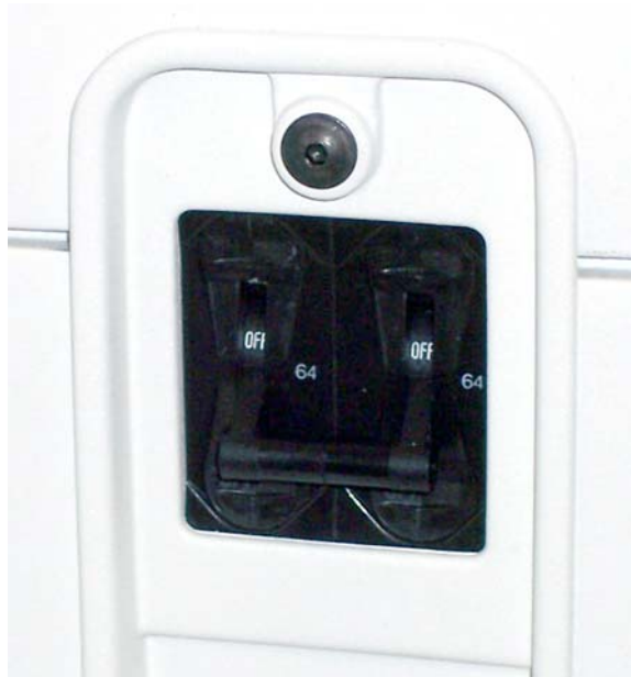
Figure 1-3 Circuit breaker (E2) in OFF position
