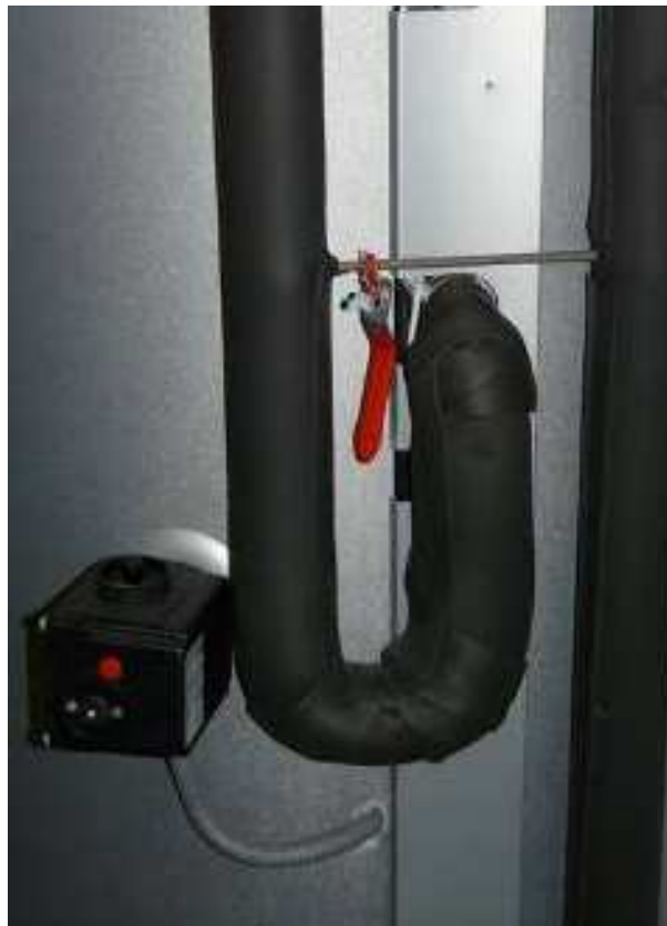
Figure 2: Pipe connection with thermo-siphon heat trap [[3]]
