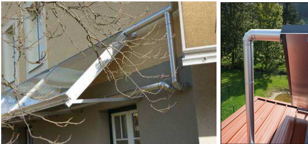
Figure 5: External pipe insulation good quality of insulation and protection
