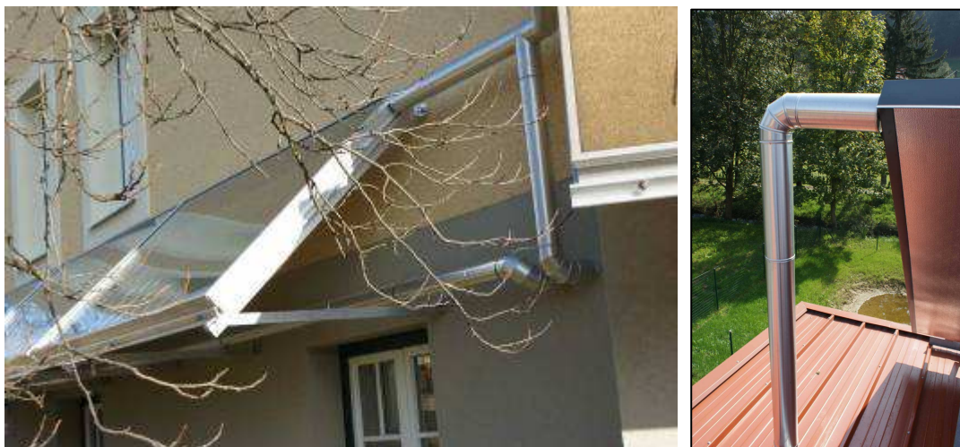
Figure 13: External pipe insulation good quality of insulation and protection
