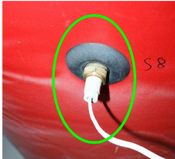
Source : AEE INTEC / Austria Figure 4: Temperature sensors fixed correctly [[3]]
