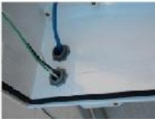
1) Pull wires to final installed length.
