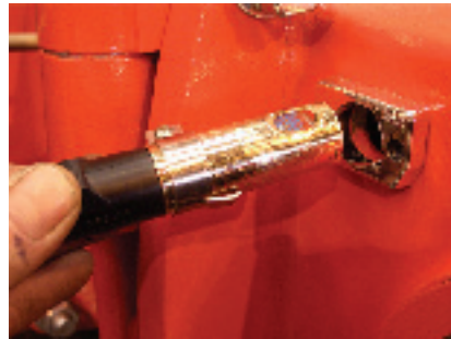
FIG. 17 TYPICAL FLAME SENSOR REMOVAL
