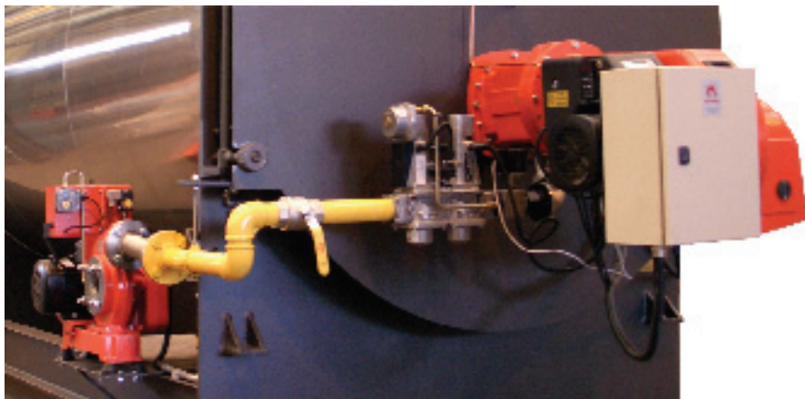
FIG. 9 GAS BURNER INSTALLATION (installation will change with the type of burner fitted)
