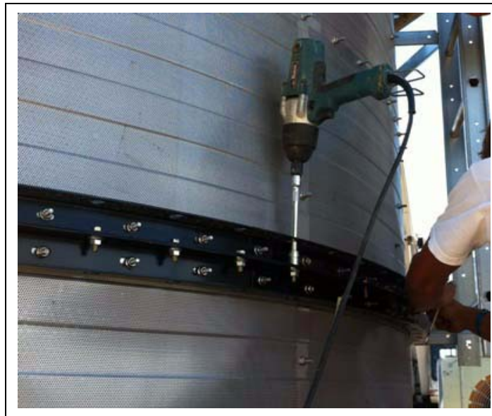
Figure 10L Connecting Dryer Sections on Outside
