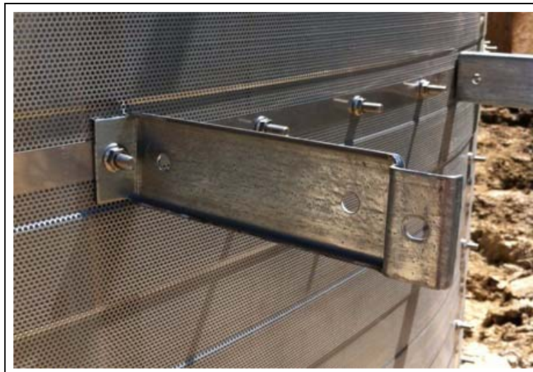
Figure 7C Ladder Brackets - Identify location on each module and surrounding equipment considerations.
