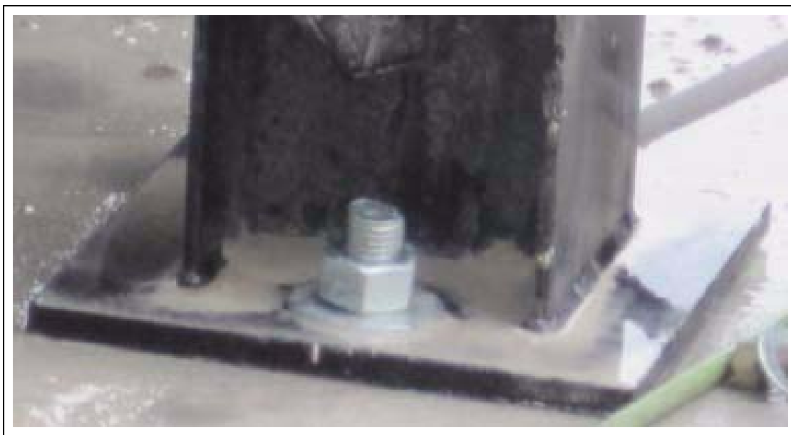
Figure 5A Anchor Bolts Sunk - No More than 3" Remains above Plate
