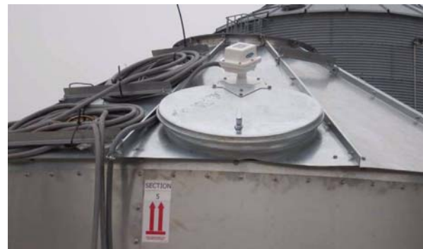
Outside view - Access port installed with decals in place.
