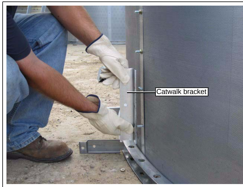
Figure 8R Attaching catwalk bracket to dryer module.
