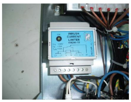
Figure 5-18 Inrush connected
