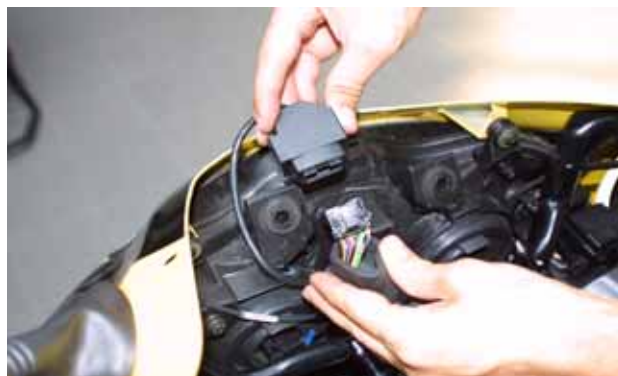
Figure 13: Wiring installation – particular of AMP connector
