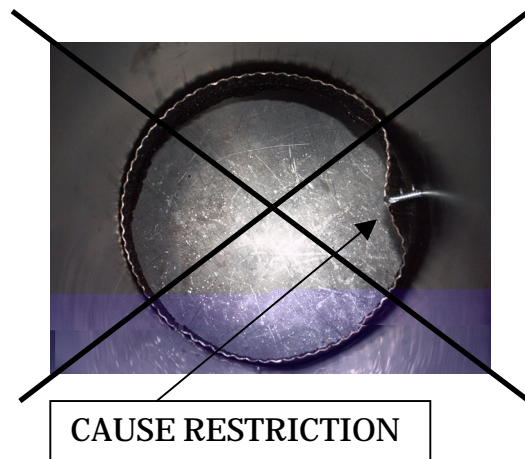
IMPROPER INSTALLATION
