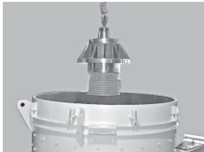
Lower rebuilt pedestal into crusher
