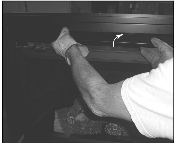
Figure 14.9 Installing Hood
