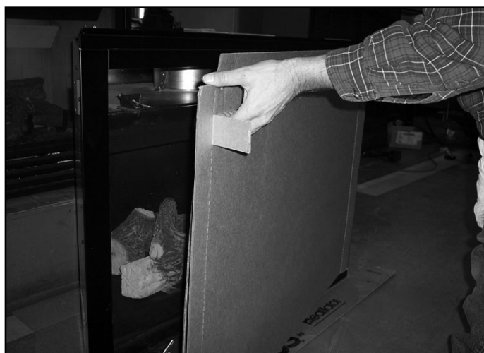
Figure 14.3 Lift up on Screen
