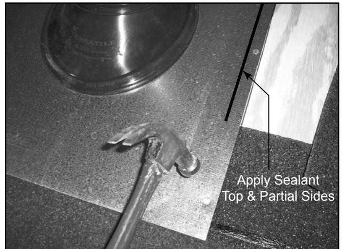
Figure 10.20 Slide Flashing Down, Secure & Apply Sealant
