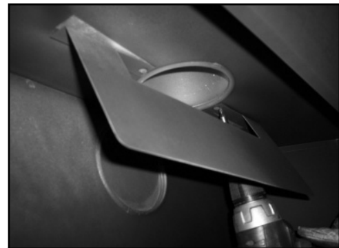
Figure 7.7b Remove Flue Visor
