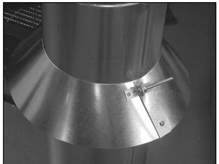
Figure 10.24 Assembling the Storm Collar Around the Pipe
