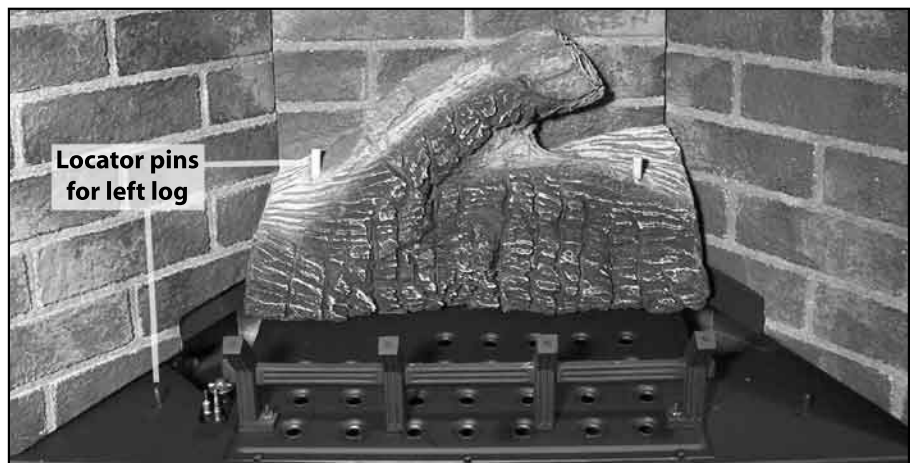
Figure 34. First Stage Log Set Installation.
