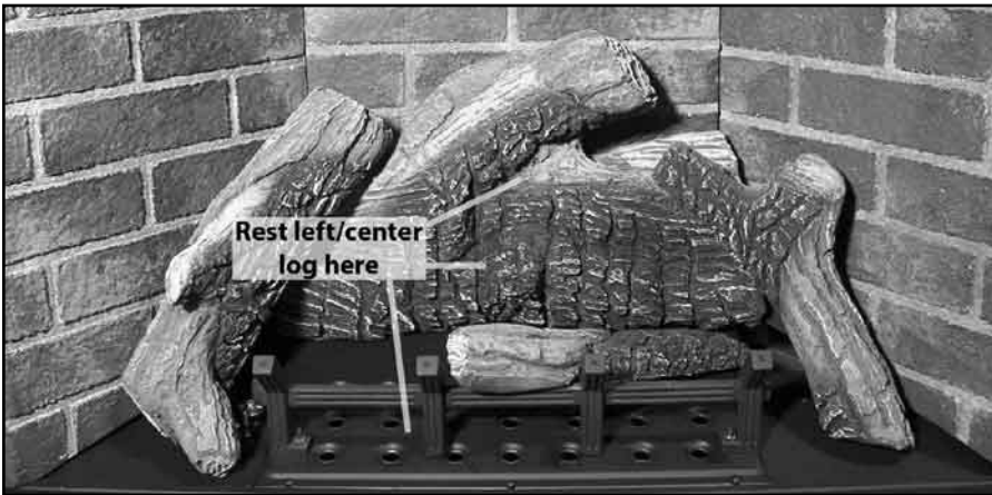
Figure 37. Fourth Stage Log Set Installation.
