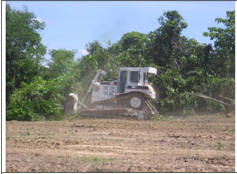
Figure 30: All top vegetation is removed by machine (bulldozer)
