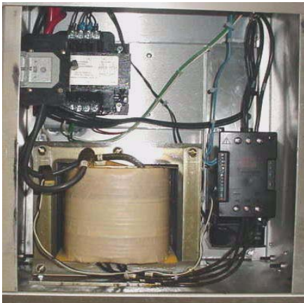
FIG. 4: Completed Installation - H-20/35 Pro
