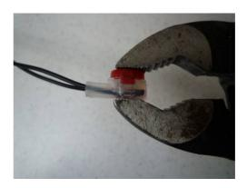
Make sure the two black wires remain fully inserted to the back wall of the connector.
