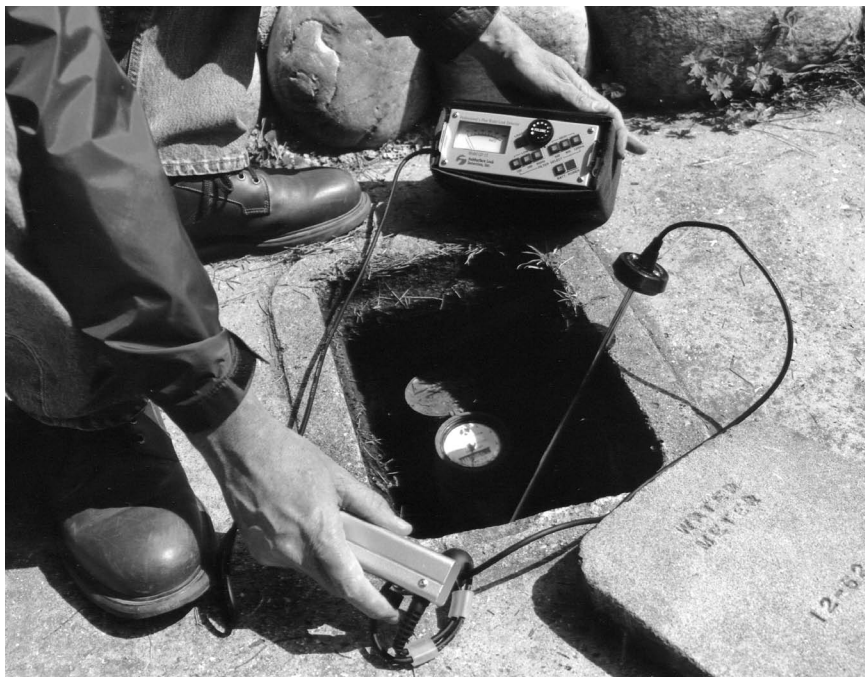
Figure 4-8 Leak Survey at a Meter
